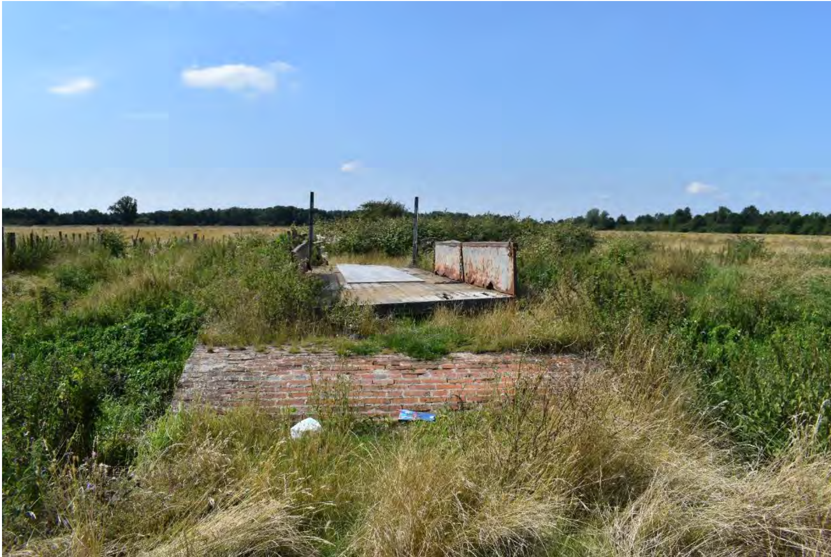
Plate 15: View of the Post Medieval bridge (facing SSW)
