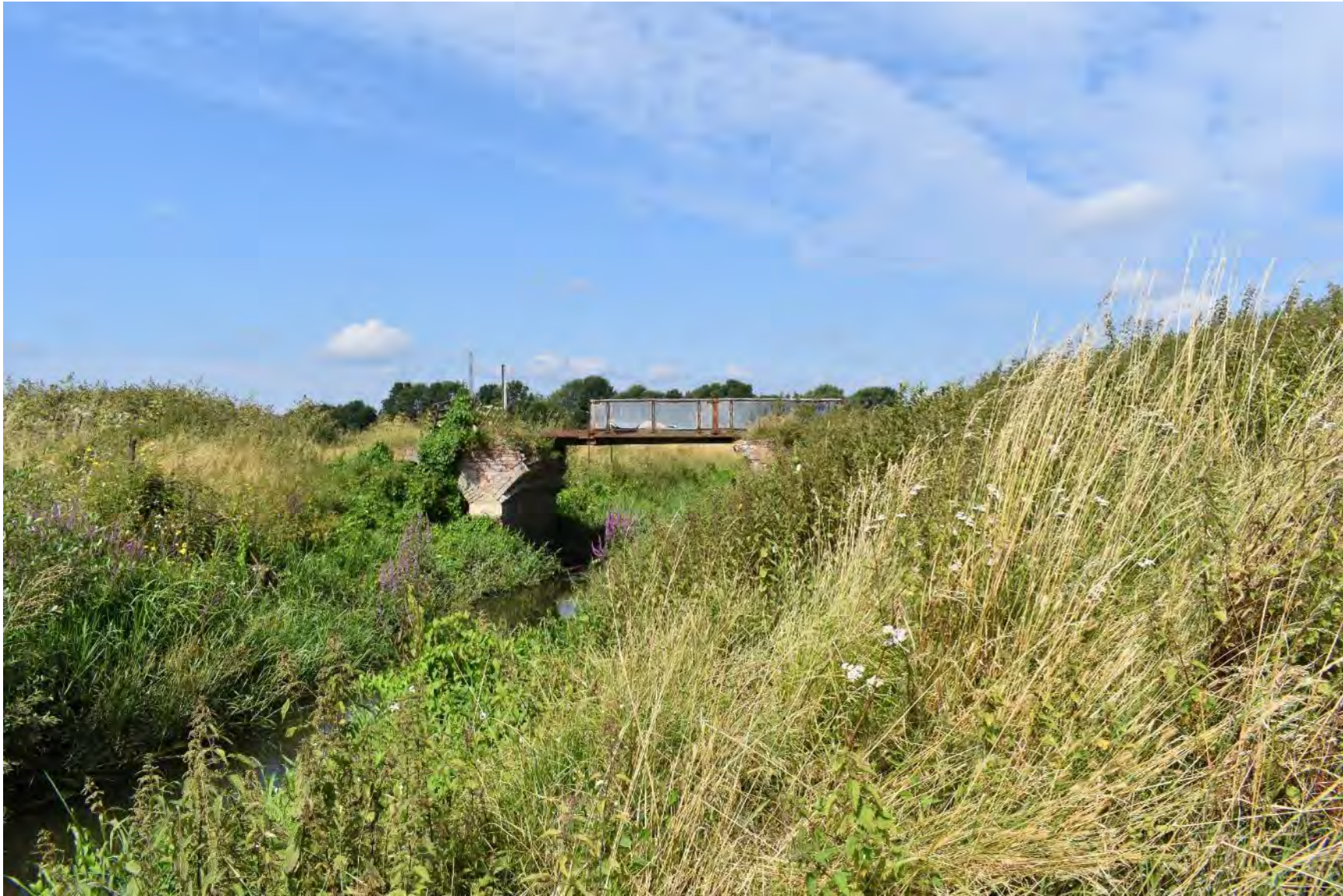
Plate 14: View of the Post Medieval bridge across the East Stour (facing WNW)
